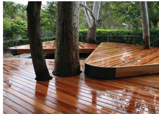
Spotted Gum Timber Decking around existing tree
