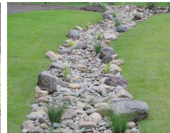
Dry creekbed - local stone and native wetland plants
