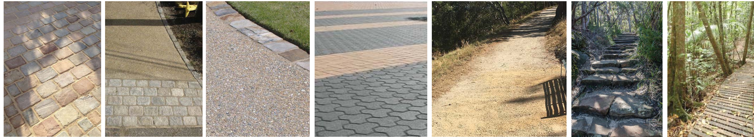
Sandstone cobblestones Cobblestone apron Exposed ag. path - Hanson Imagecrete 'Derwent' Permeable concrete paving Crushed limestone gravel path Stone steps Timber bridge
