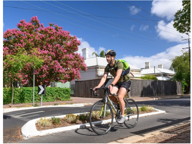
Street slowing using planted pinch points with bike by-pass (Unley, South Australia)
