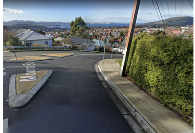
Steep and misaligned kerb ramps, slip lanes, and obstructed footpath at Mount Stuart Rd / Mellifont Street intersection
