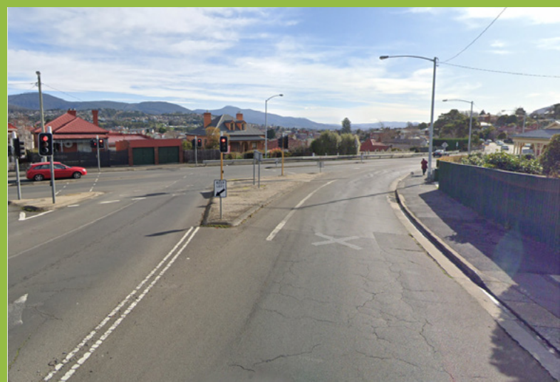
Wide streets and inappropriate intersection geometry encourages high speeds
