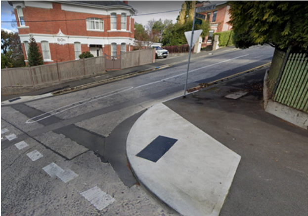
Steep kerb ramps at Elphinstone Rd / Mount Stuart Rd intersection
