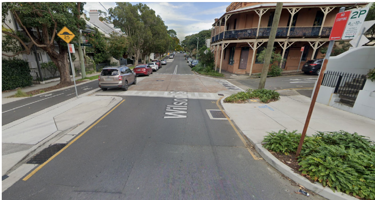
Wilson Street in Eveleigh, NSW, accommodates traffic, on-street parking and a bidirectional bike path in the same road reserve width as Augusta Road (20m)
