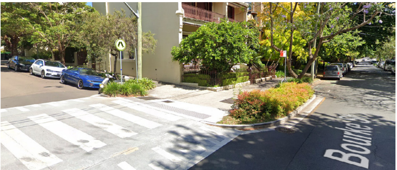
Kerb extension and continuous footpath treatment (Surry Hills, NSW)
