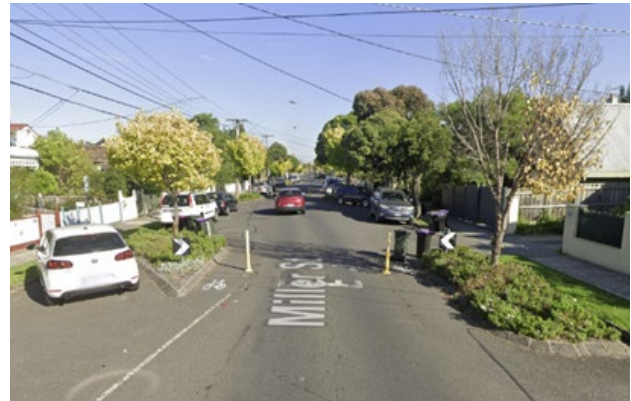
Figure 20. Example of a negotiated slow point also serving bus services. Miller Street, Fitzroy North, Victoria.
