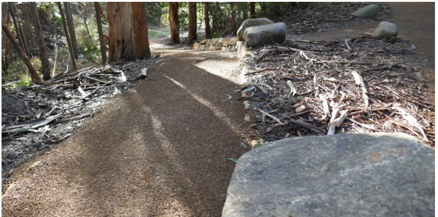
Completion of the new walking track at Salvator Rosa Glen Creek.
